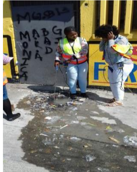
Leak Detection in progress
